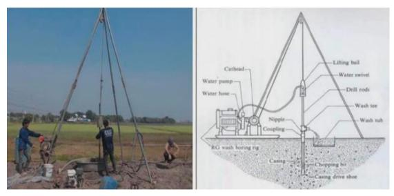
**d. Excavation by drilling:-**This method is used especially in areas with hard soil and rocks ,the soil and rocks are fragmented By continuously hammering the bottom of the hole with a drill bit, and water is passed over the loosened soil. This method can be beneficial in soils containing layers by changing the rate of drilling speed
