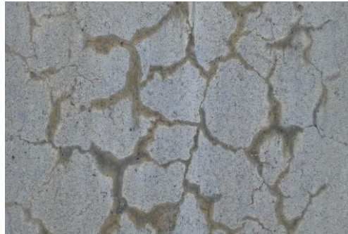
alkali aggregate reaction
