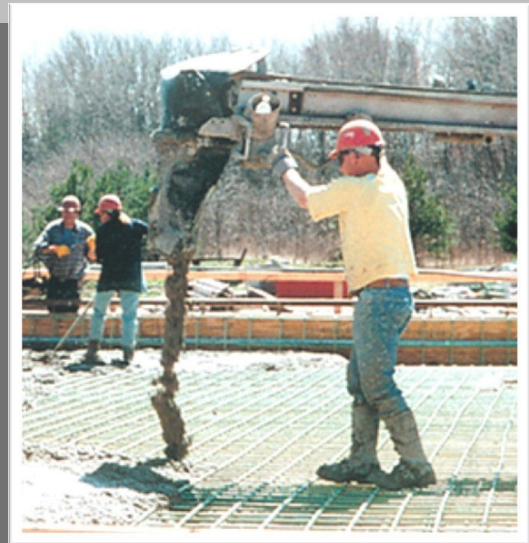
Placement with Conveyor Belt
