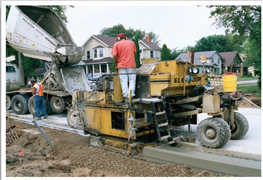
Placing and Finishing Concrete
