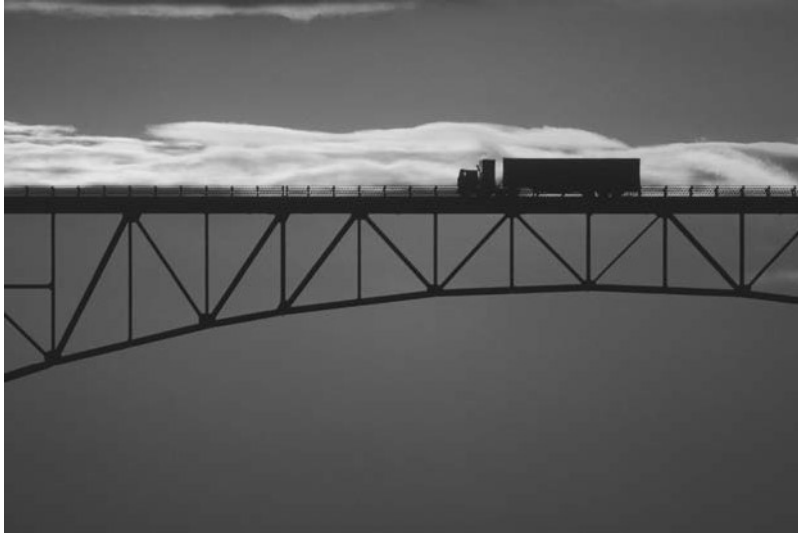
Fig. 1.9 This bridge truss consists of two-force members that may be in tension or in compression.
