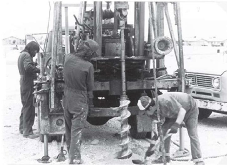
Figure 3-3 Soil drilling using a continuous-flight auger .
