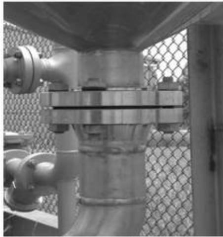
Stainless steel nozzle & welded neck flange (Std ANSI 150)
