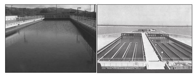
The settling tank is designed so as to remove the settled water from the tank without carrying away any of the floc particles. In ideal sedimentation process, the average velocity of the water is equal to its flow rate divided by the area through which it flows:
