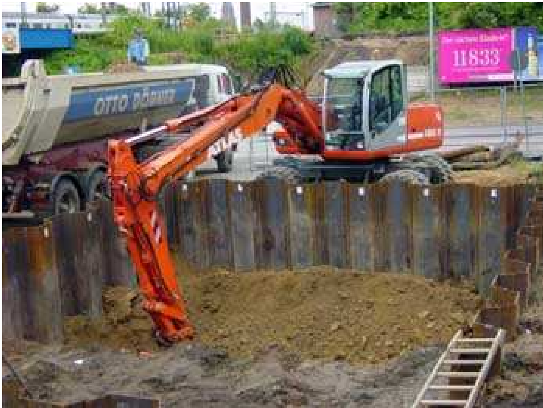
Fig.7 Mobile Wheeled Excavator
