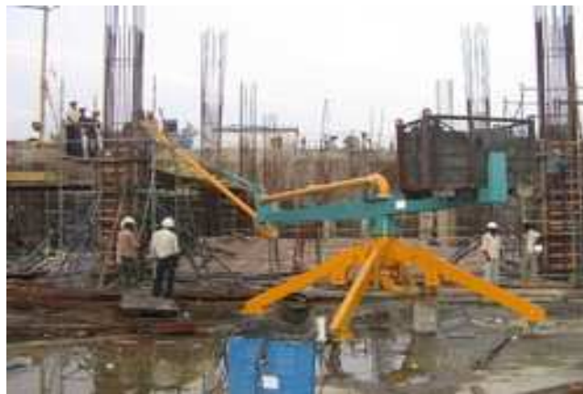
Fig.5 Concrete Distributor
