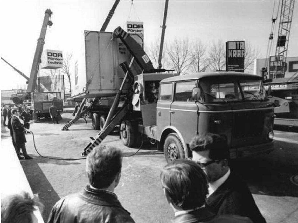
Fig.3 Side lift Crane
