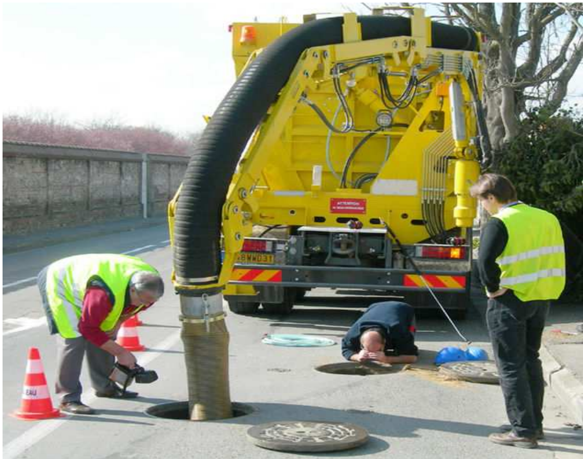
Fig.14 Cleaning out a sewer manhole
