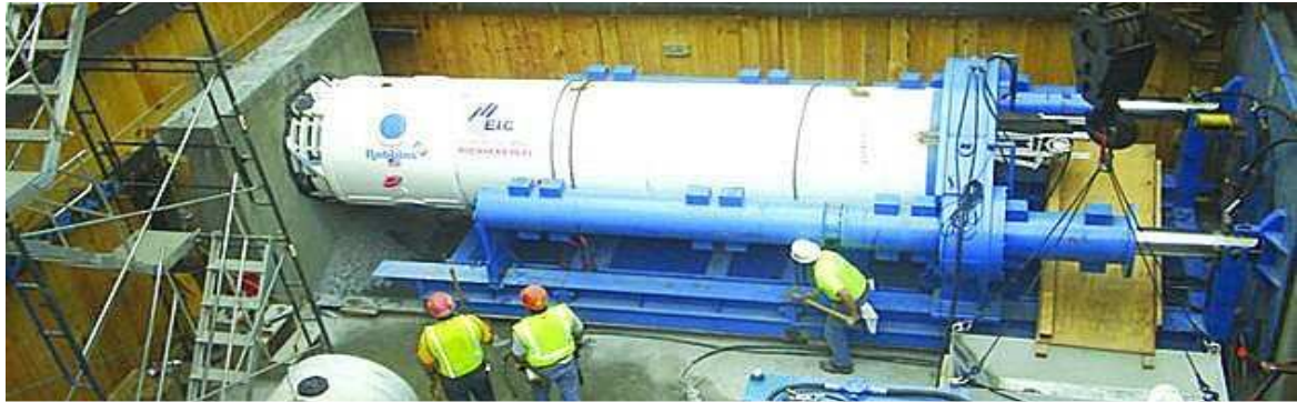
Fig. 6 Microtunneling Boring Machine
