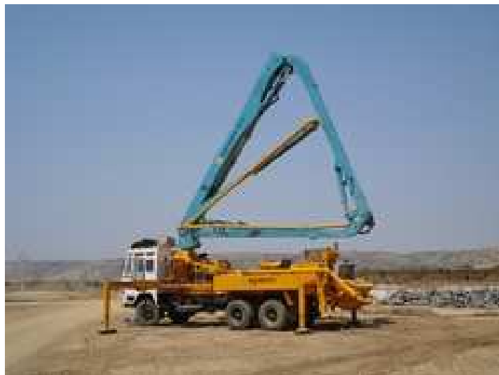
Fig.1 Concrete boom pump
