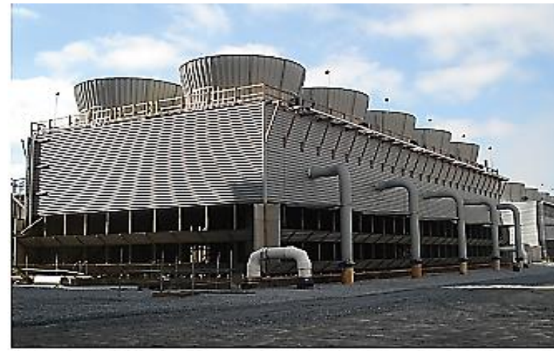
Field-erected (FEP) cooling tower – induced-draft counterflow cooling tower
