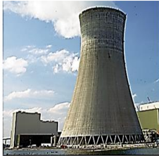
Natural-draft cooling tower — field-erected (FEP) counterflow cooling tower
