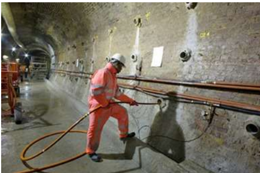
Pic. (47): Injection Grouting in to concrete wall tunnels
