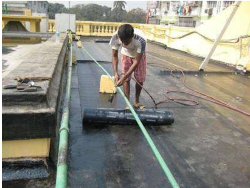
Pic.(42): Surface treatments to limit corrosion by reducing the existing moisture level in the concrete.
