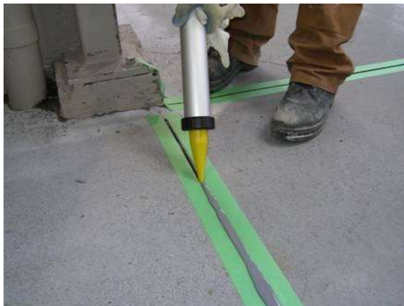
Pic. (45): Injection of joints with flexible material
