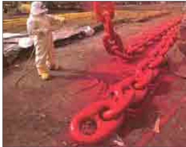
Protective colour coatings are added to make components it corrosion resistant. Corrosion if not taken care can magnify other stresses.
