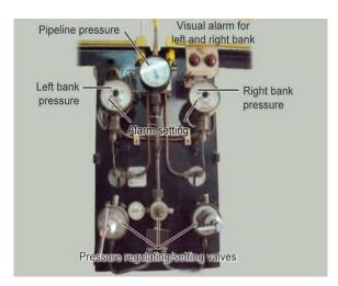
**Note1:** Manifolds are two banks (one right sided bank and one left sided bank) Large cylinders (e.g. size J each with 6800 L capacity) are usually divided into two equal groups, primary and secondary. The number of cylinders depends on the expected demand.
