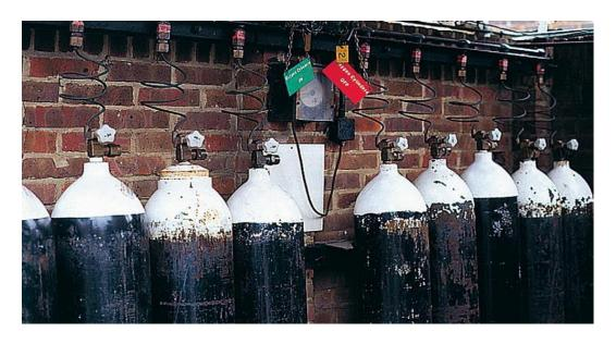
**Note2:** All cylinders in each group are connected through non-return valves to a common pipe. This in turn is connected to the pipeline through pressure regulators.
