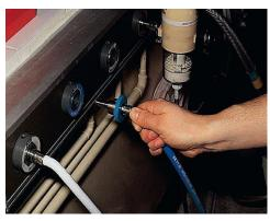
The size of the pipes differs according to the demand that they carry. Pipes with a 42 mm diameter are usually used for leaving the manifold. Smaller diameter tubes, such as 15 mm, are used after repeated branching.
