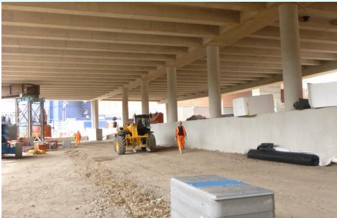
Flat slab with drop panel and column head
