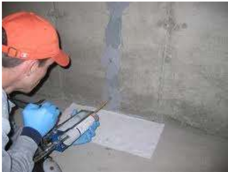
Pic. (36): Epoxy injection for Concrete Crack Repair in basement wall
