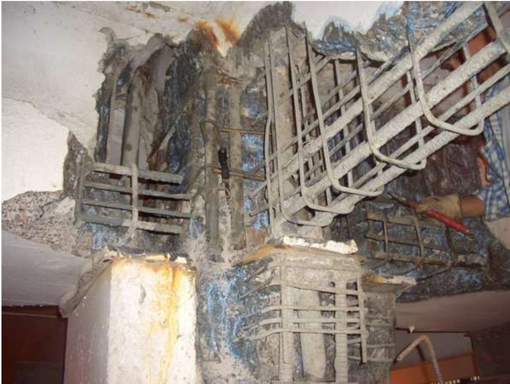
Pic. (35): Preparation of surface for replacement concrete
