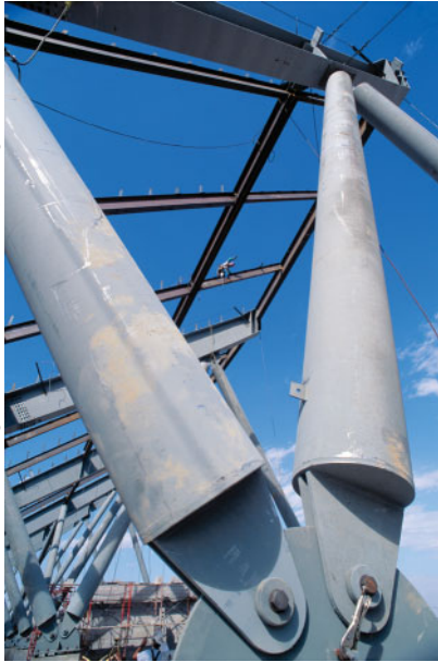
The structural elements in the foreground transmit concentrated forces to the brackets at both ends.
