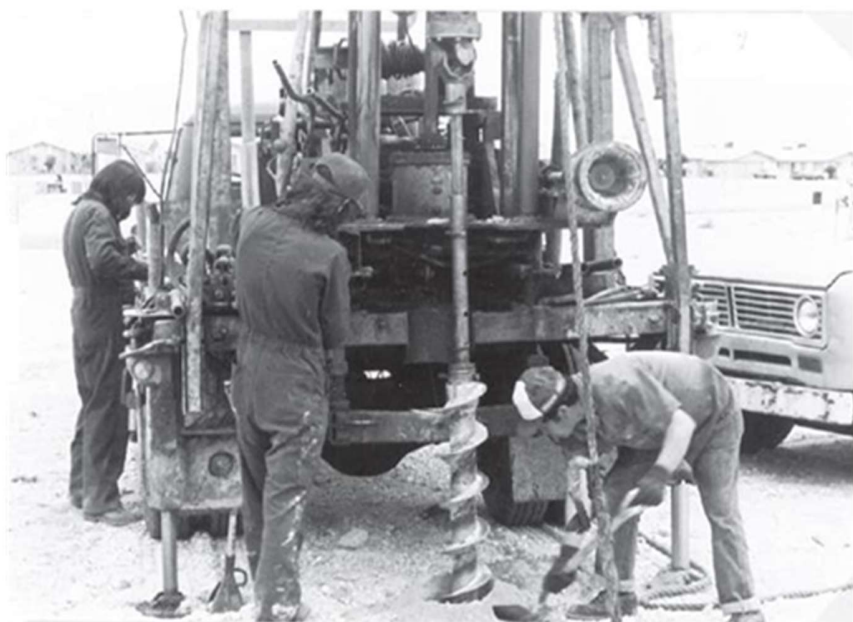
Figure 3-3 Soil drilling using a continuous-flight auger.
