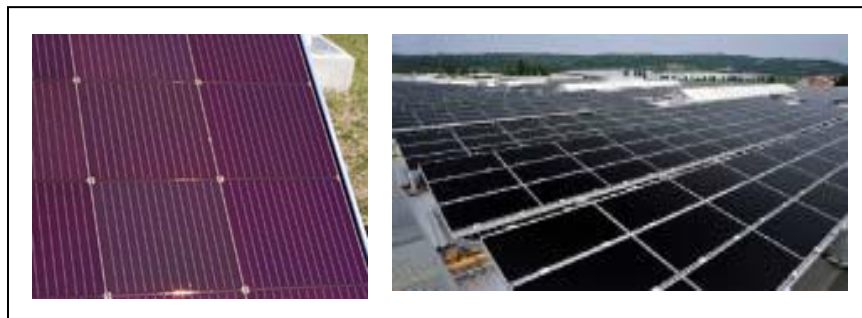
Figure 3.6: Left hand and right hand view of a thin film Cadmium Telluride
