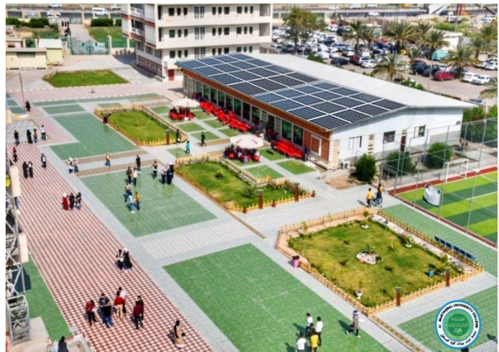
Figure 4. Roof Mounted Solar Panels on the administration building and the main restaurant.
