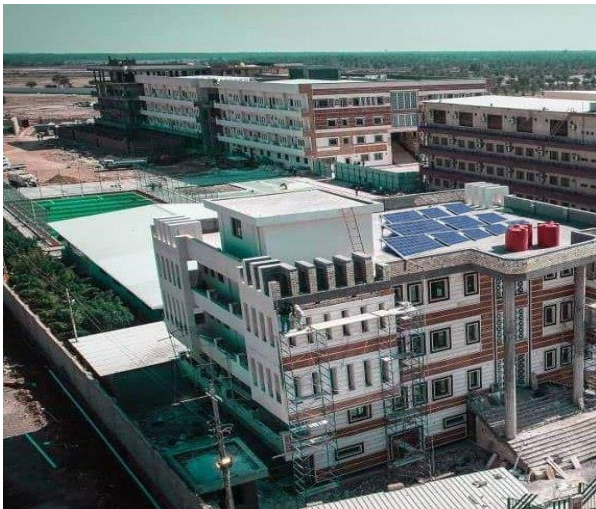
Figure 4. Roof Mounted Solar Panels on the administration building and the main restaurant.
