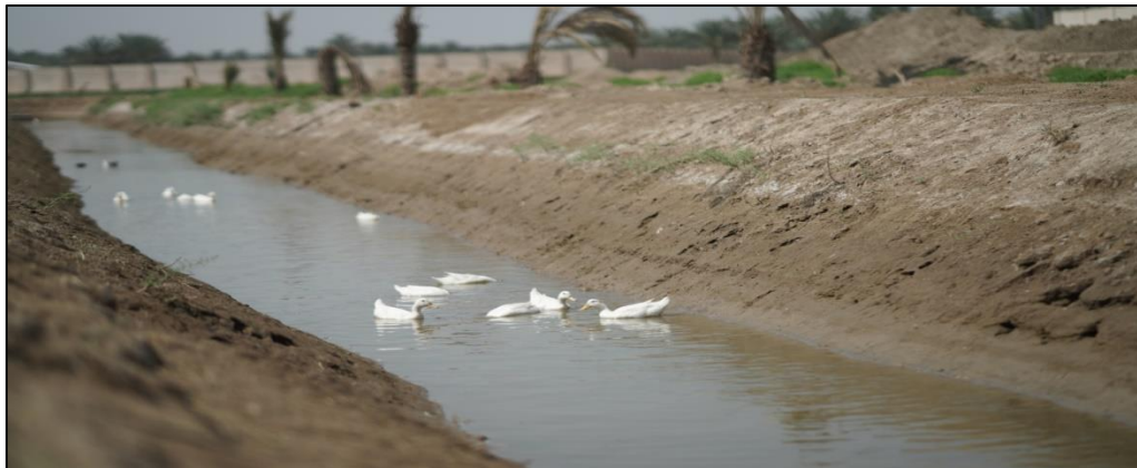
Figure 3: Irrigation channel inside Al-Mustaqbal University
