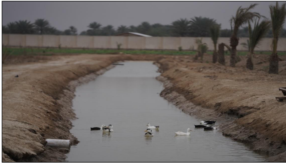
Figure 2: Irrigation channel inside Al-Mustaqbal University
