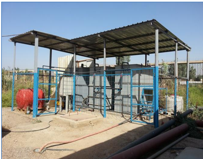
MBBR technique for wastewater treatment
