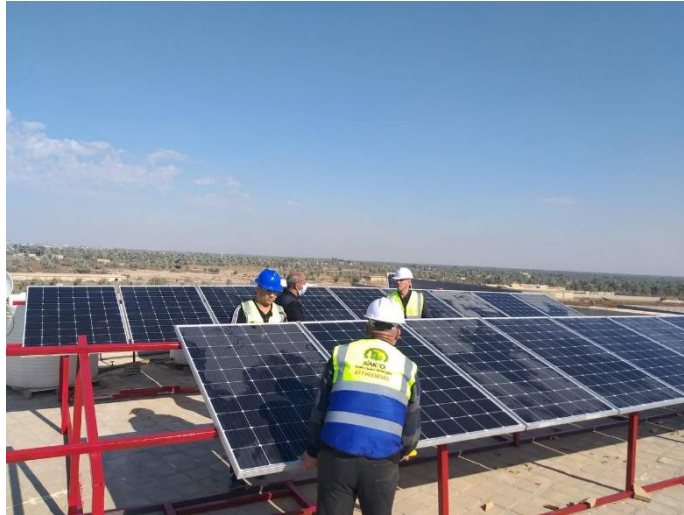
Figure 6. Installing solar panels on the medical building
