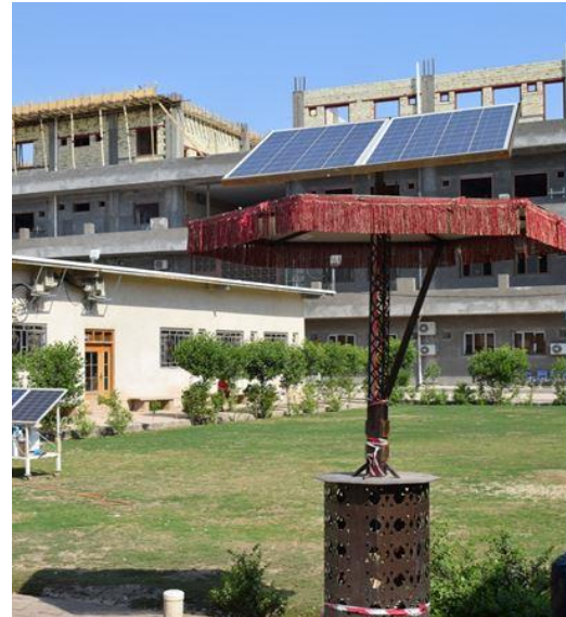
Figure 8. Utilization of Solar Panels for Multi-Purpose such as Device Charging
