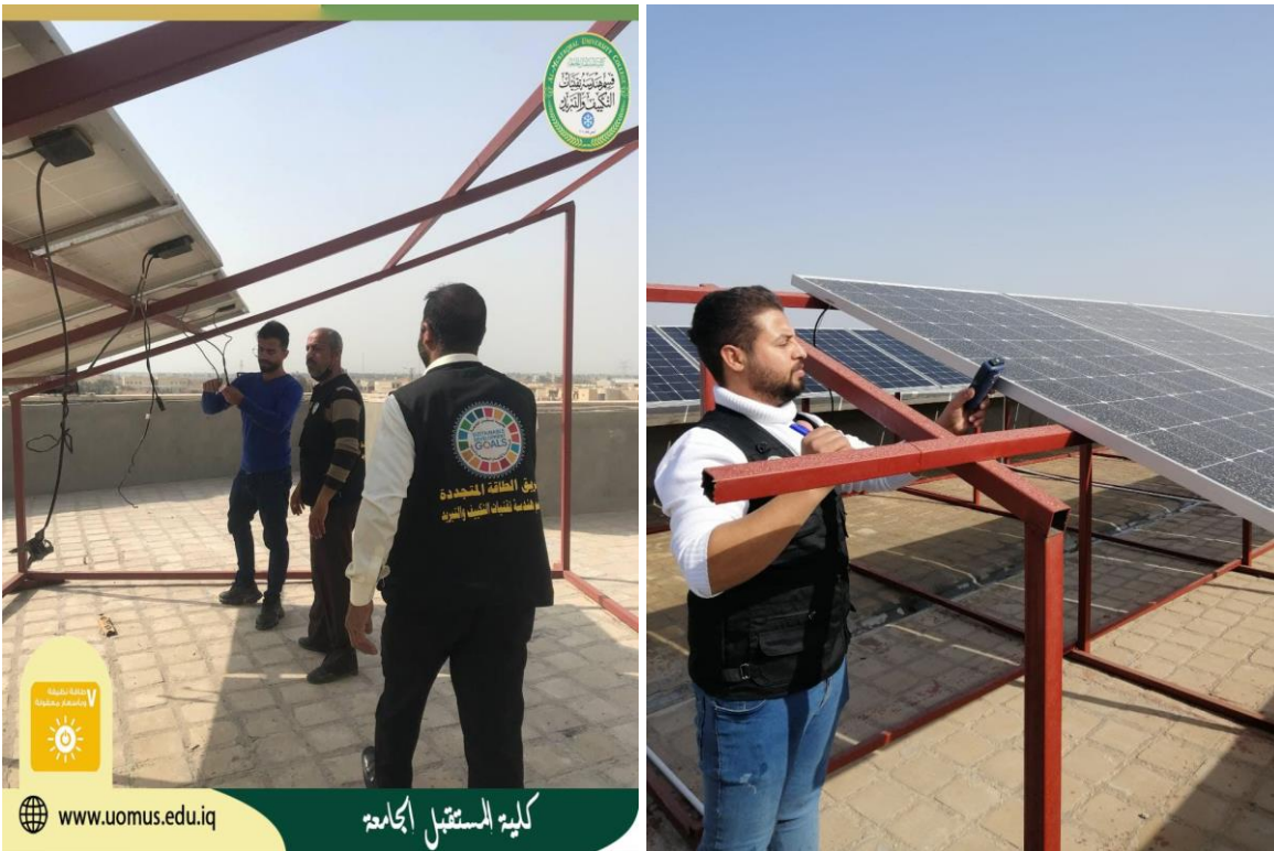
Figure 1. Installation of solar panels on the roofs of the buildings
