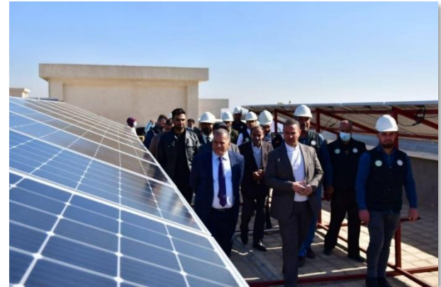
Solar cells that installed by the staff of the Air Conditioning and Refrigeration Technologies Engineering Department
